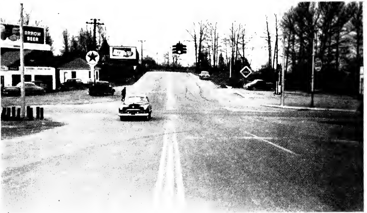
WIDENING AND RESURFACING INTERSECTION OF U.S. ROUTE 301 (CRAIN HIGHWAY) AND MD. ROUTE 214 (CENTRAL AVENUE), TO PROVIDE ADDITIONAL TRAFFIC LANES
